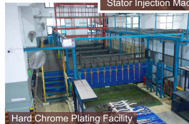
Hard Chrome Plating Facility
