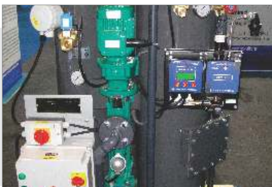
Roto Pump feeding oily water on OWS
