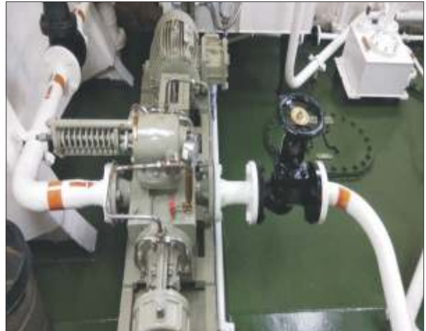
Fuel Oil Transfer - Coast Guard Patrol Vessel, Goa Shipyard, India
