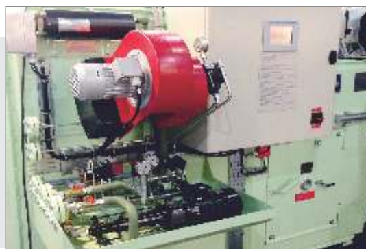
Roto Pump feeding dirty oil for incineration
